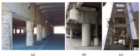
In particular, several bridge columns and beams damaged by steel corrosion along a major highway in Toronto made the bridge seriously deficient [Figures 12(a) and 12(b)] (Homam et al., 2001; Kharal and Sheikh, 2018; Sheikh and Homam, 2004; Sheikh and Yau, 2002). An industrial structure was also studied which was found to be shear critical
